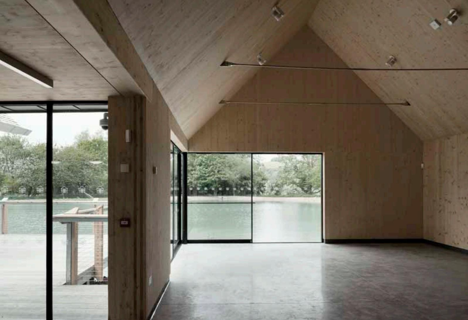
The buildings were conceived as two primary elements – green oak frame and Cross Laminated Timber (CLT) – and aim to provide knowledge and understanding of modern forms of construction, making clear references to their historical counterparts whilst marrying traditional and modern technology and materials. Both of the entrance buildings are designed and built as solid timber buildings.
