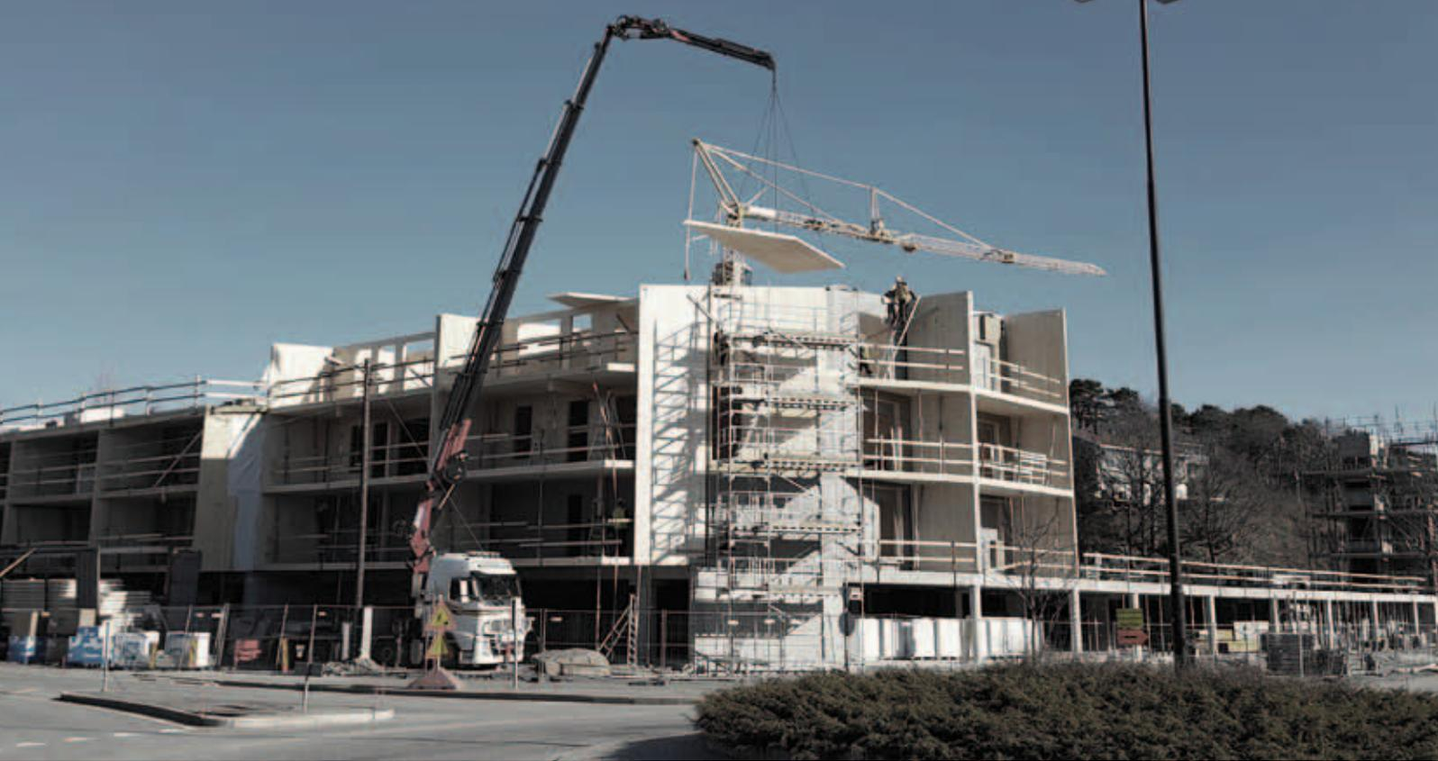
A total of 8,500 m<sup>2</sup> of CLT panels make up the 2,850 m<sup>2</sup> of apartments in stages 1 & 2. All the buyers had the option to choose from exposed wood panels or gypsum-clad walls inside the apartments, and all of them chose the visible wood option. 50% of wall surfaces are now exposed wood inside the apartments.
