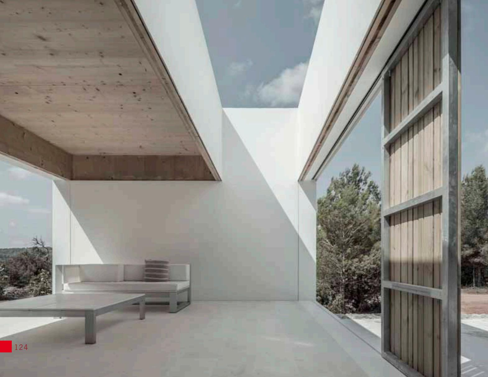
All the facades are ventilated and breathable, featuring two different solutions and finishes: the transverse, opaque facades in contact with the dry stone walls that contain the earth have been finished using slats of thermo-treated wood, while the longitudinal ones, where the openings and patios are concentrated, have been carried out using synthetic, large-format, mineral-based panels.
