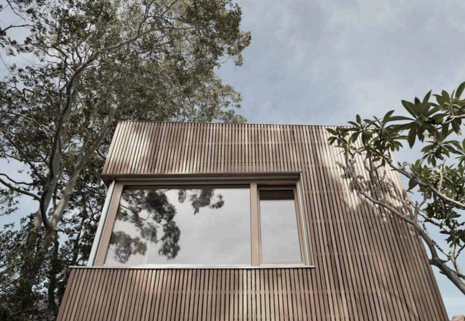
The CLT walls are externally insulated with wood fibre insulation and a ventilated cavity façade, clad in local Blackbutt timber battens and left untreated so it can naturally grey over time. The rough sawn timber façade creates the connection between the trees in the garden and the exposed timber walls of the internal spaces.
