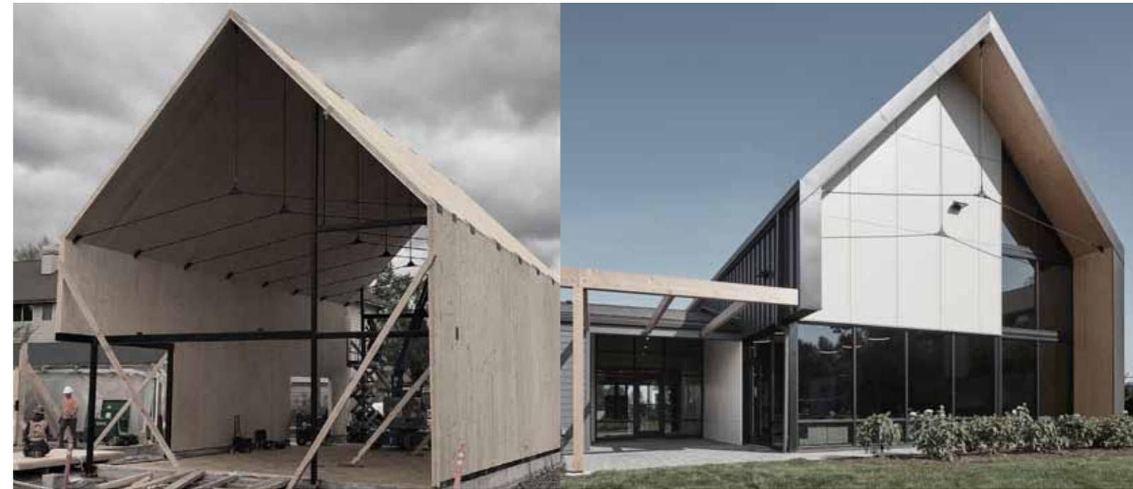
The gable forms of the two volumes were chosen for their structural capabilities and recognizable icon as a „house“. The distinct gable forms and exposed KLH® - CLT material on the interior created warm and light filled spaces.
