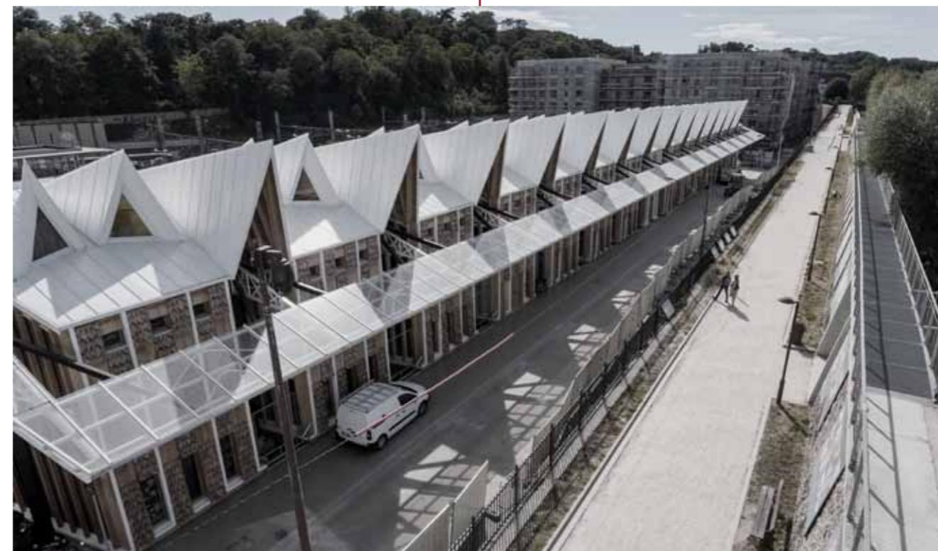
As it was decided not to use the skeleton of the former hall as a support structure, the spatial programme now circumvents this original function. The façade is suspended from supporting points. This curtain wall façade with its “folds” allows outward views and natural illumination of the offices, and separates 15 work areas each with a wooden area of 75m<sup>2</sup>.
