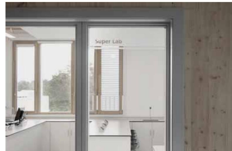
The structure is predominantly KLH® - CLT and glulam with a limited amount of steel and a concrete plinth, although the team suggest that a greater use of KLH® - CLT may have reduced the complexity of detailing and construction involving glulam elements, particularly to external walls.
